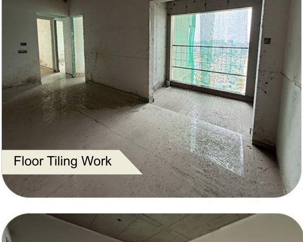
Floor Tiling Work
