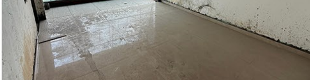
Floor Tiling Work
