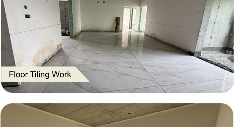
Floor Tiling Work
