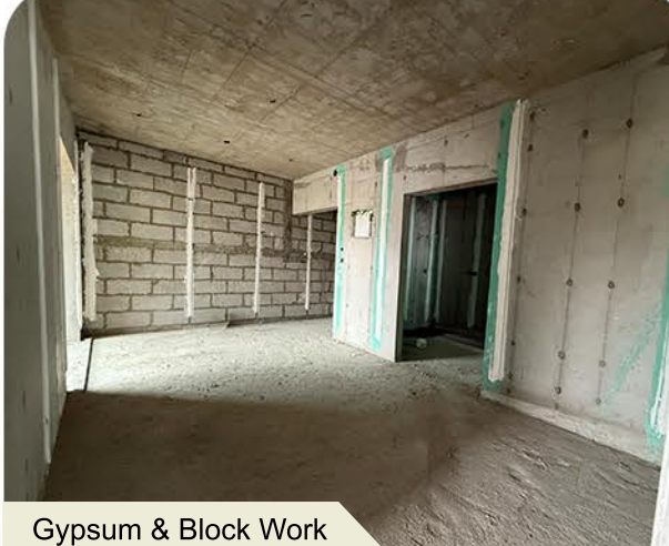
Gypsum & Block Work
