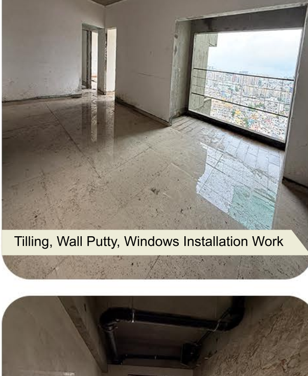
Tilling, Wall Putty, Windows Installation Work
