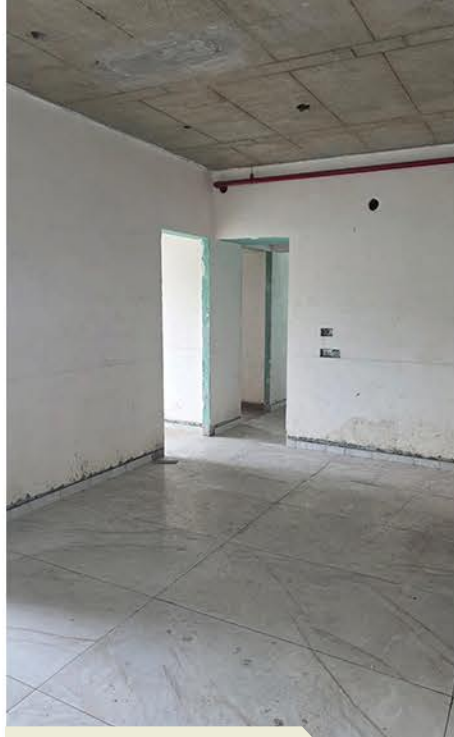
Internal Flat Flooring
