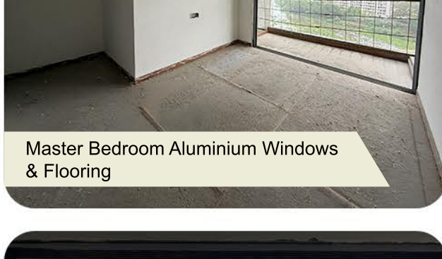
Master Bedroom Aluminium Windows & Flooring
