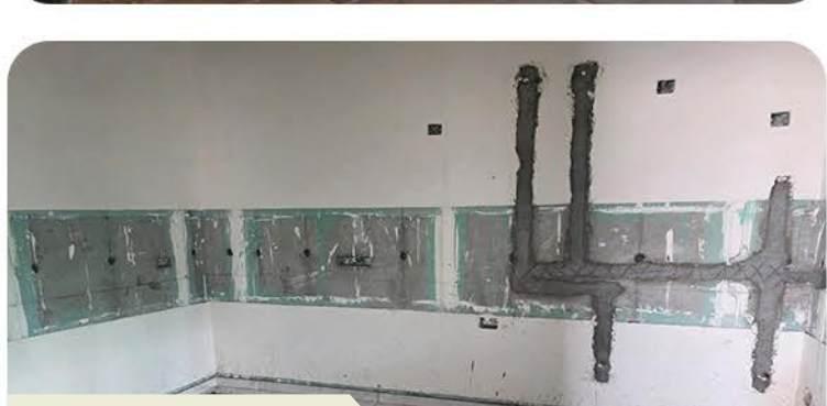
Kitchen Plumbing Work
