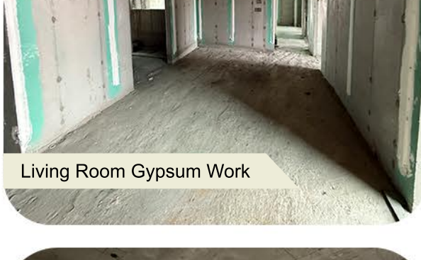
Living Room Gypsum Work
