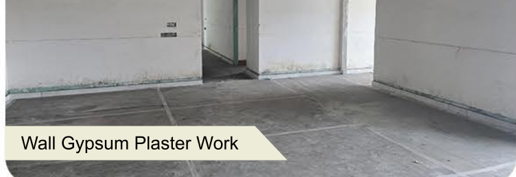
Wall Gypsum Plaster Work
