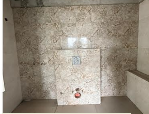
Toilet Dado and Plumbing Work
