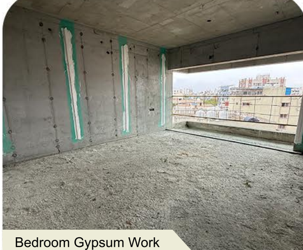
Bedroom Gypsum Work
