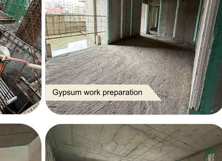
Internal tiling and wall Gypsum
