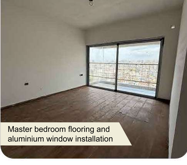
Internal flooring and painting work
