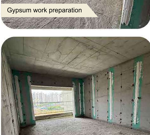
Gypsum work preparation
